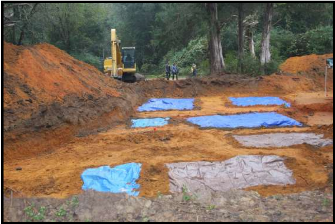
Figure 17. Burials are protected with tarps until the team can hand excavate.
