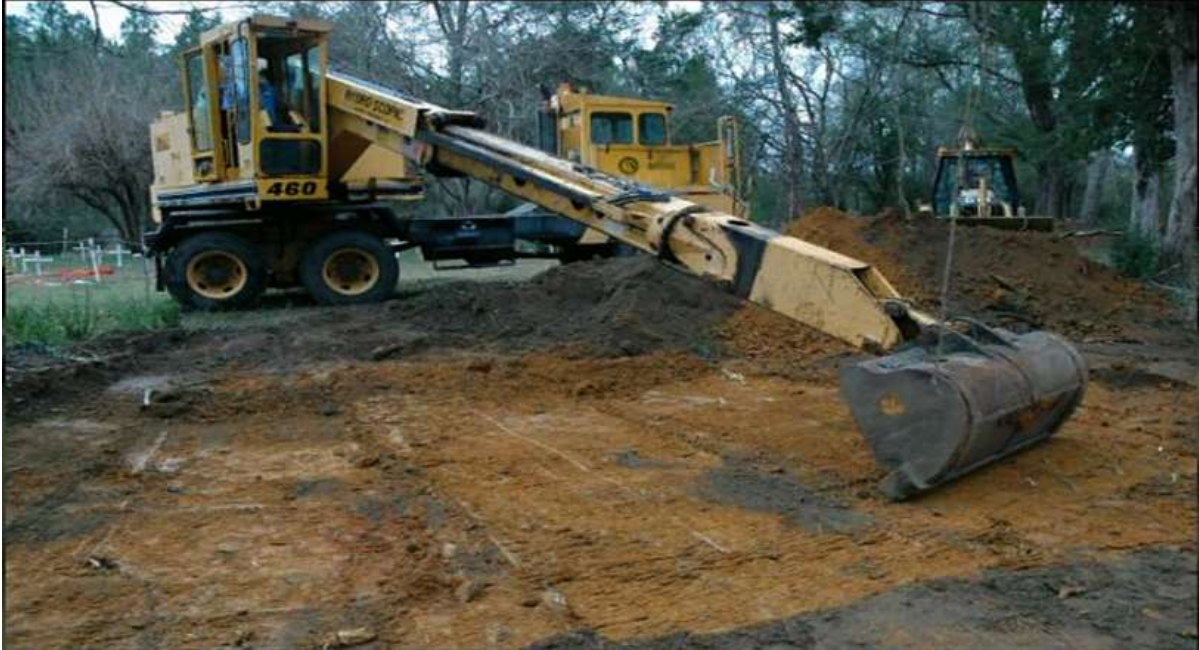
Figure 15. Heavy equipment removes the topsoil with a flat blade.
