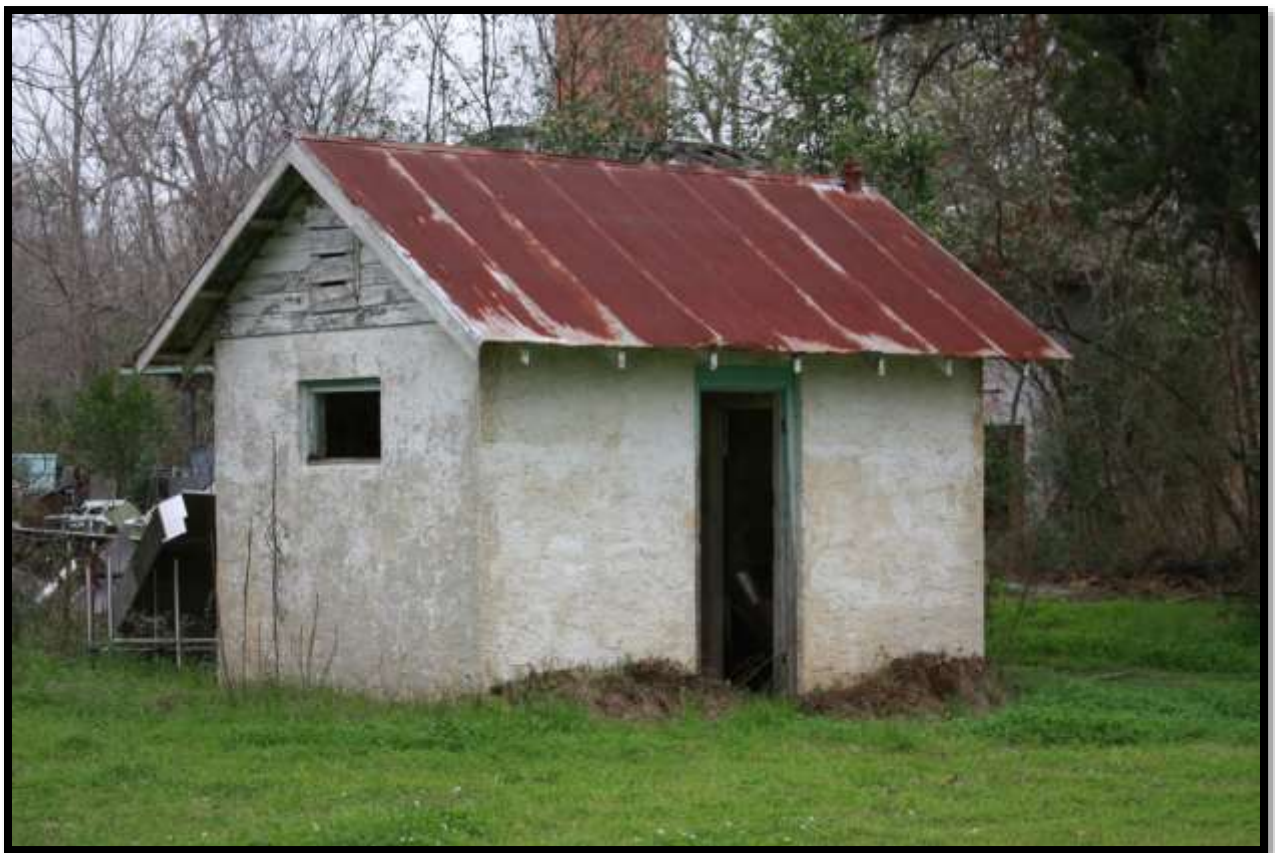
Figure 80. Former farm manager's office converted into a confinement cottage on the North School. The building had originally been constructed for storing farm goods. The interior measurements of the building are 7.0 by 10.0 feet in dimension and it is believed to be the location of the death of Earl Wilson in 1944.
